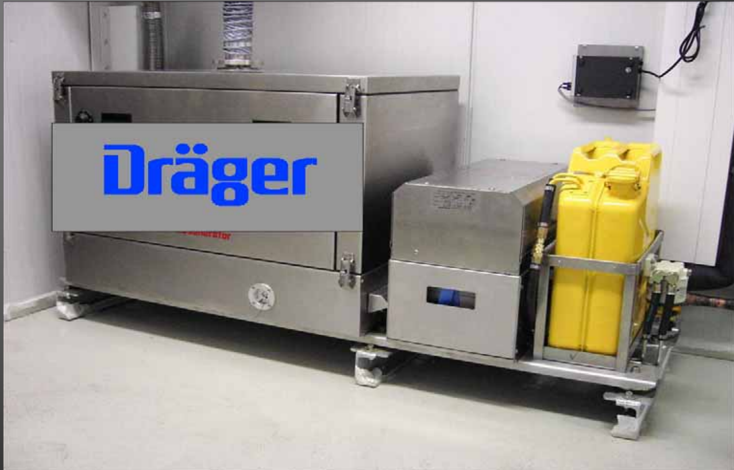
Back up electrical generator
