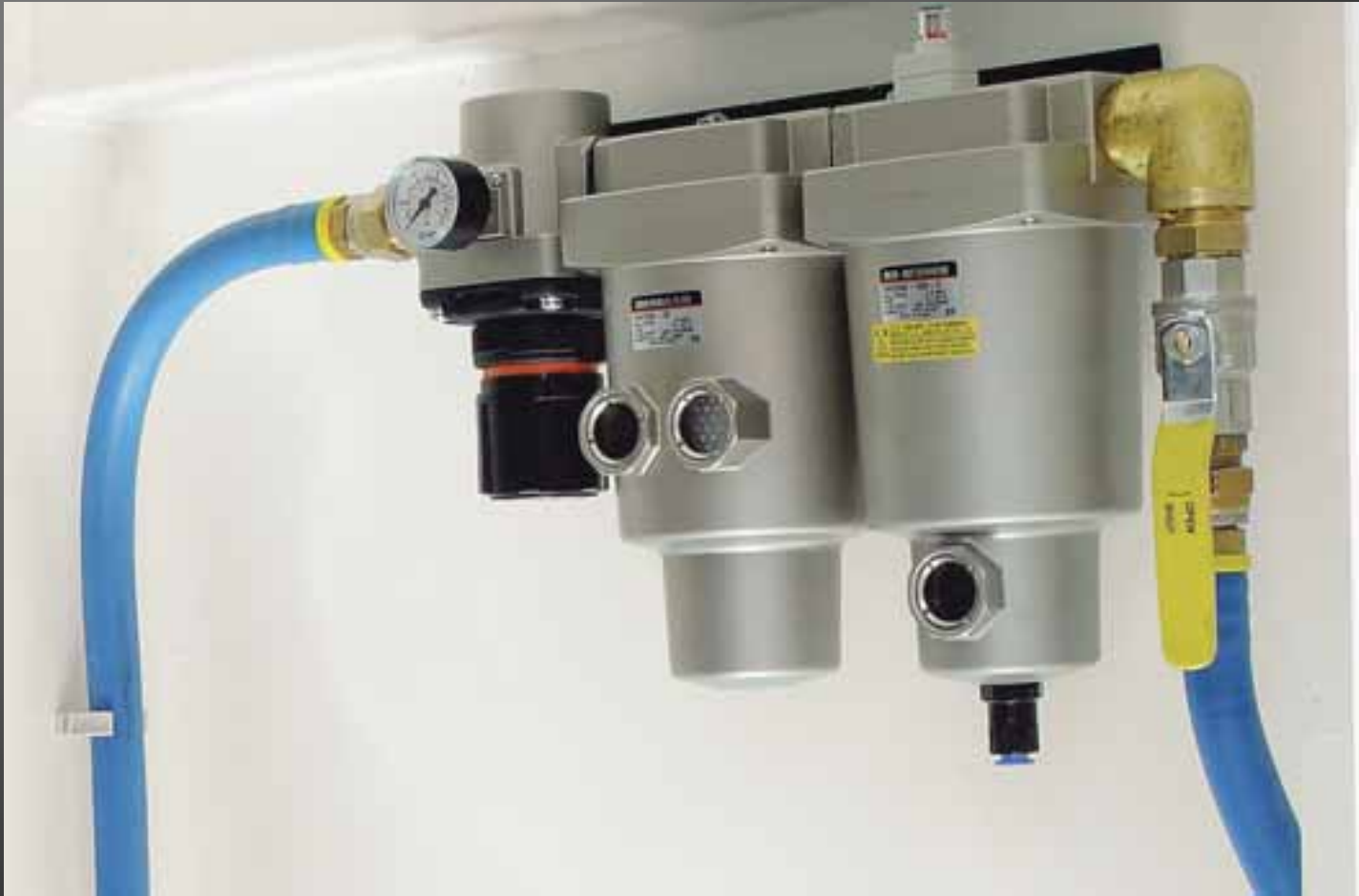
Mine Compressed Air Supply and Filter Assembly
